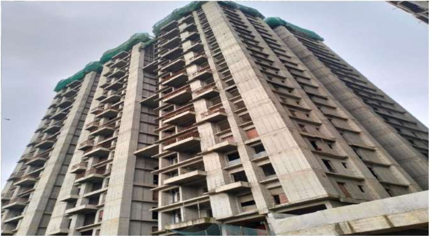
BLOCK-1 ROOF CASTING COMPLETED
